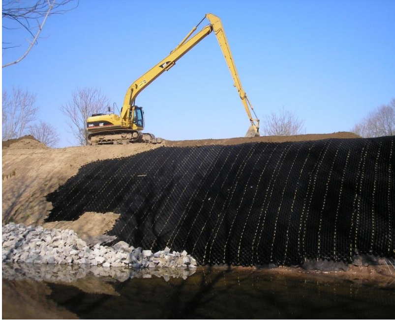
Wissahickon Creek Streambank Geocell & Rip-rap Installation
