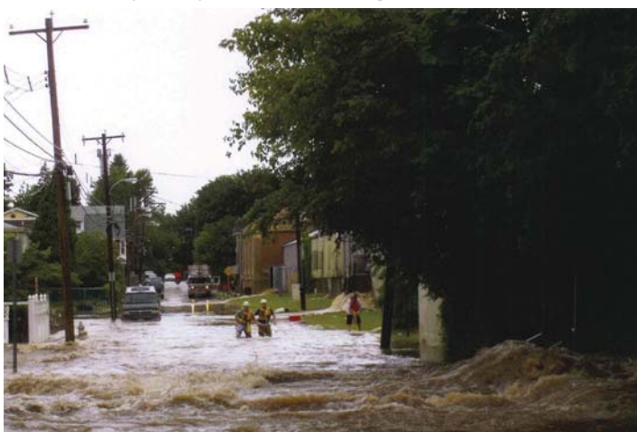
Figure 4.5 Flood waters overflow Rose Valley Creek sluiceway during Tropical Storm
