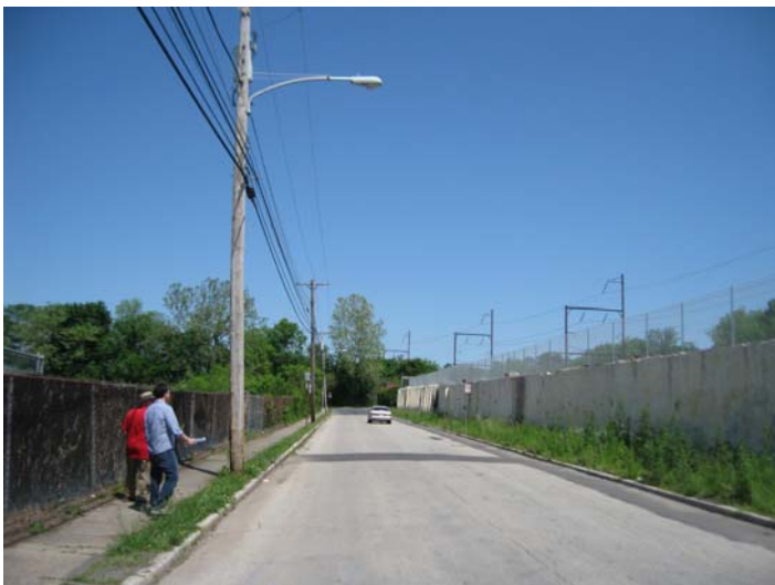
Figure 2.17 West Maple St. looking West with a Vacant building pad to the right.
