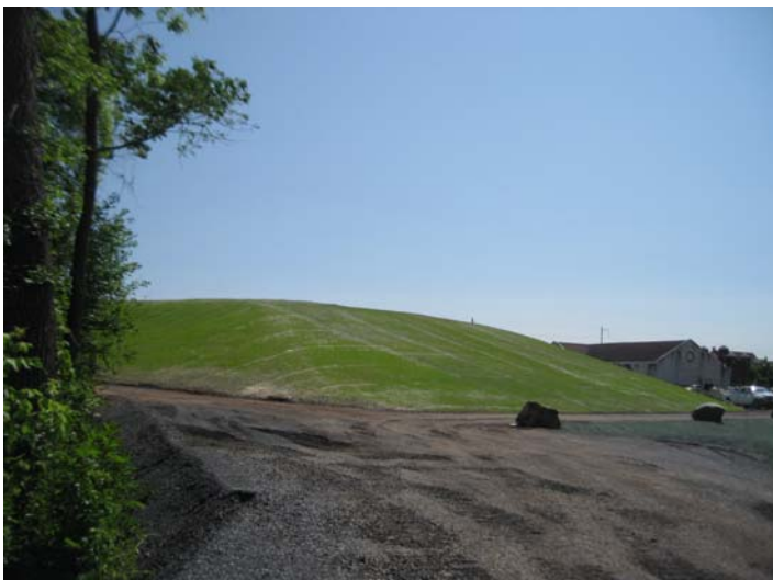
Figure 3.3 The “Pile” site after EPA emergency response work.
