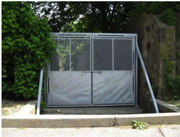
Figure 4.7 New flood gate installed on Rose Valley Creek at West maple Street following Tropical Storm Lee.
