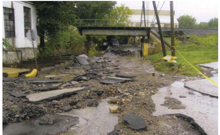
Figure 1.8 Damage to Tennis Ave after Tropical Strom Lee in 2011.
